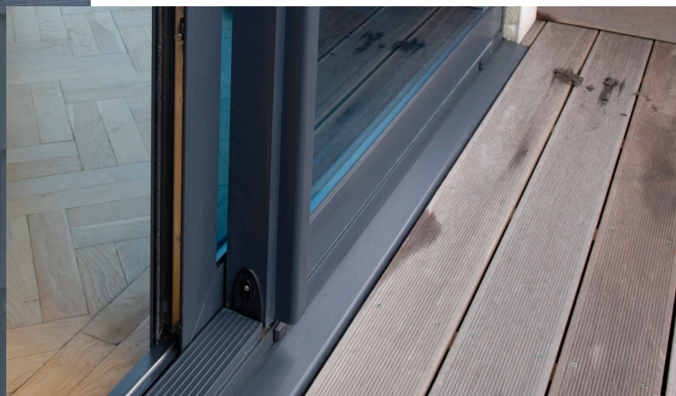
Twin Track Sliding Doors
